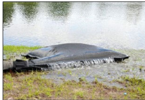
Plate 2-2 Silt Bag with water being pumped through
