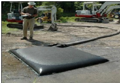
Plate 2-1 Silt Bag under inspection
